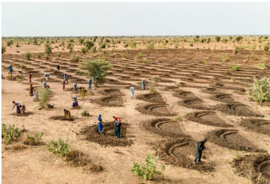
Half-moon cultivation consisting on degraded soils in an arc-shaped earth embankment in order to promote the capture of runoff and the penetration of water on degraded soils. North Senegal, © WFP, Evelyn Fey
